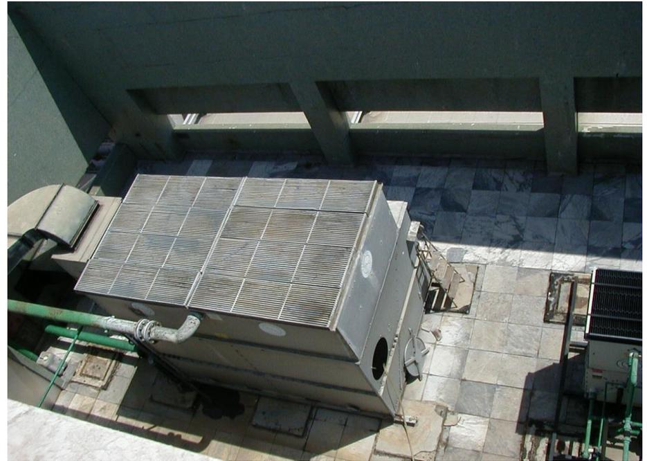
Figure 1.1 Induced draught counterflow cooling tower
